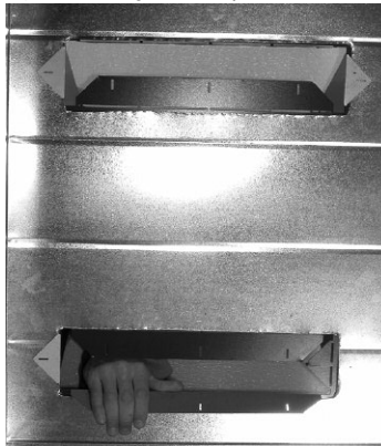
figure 2.3b - Unfold the ducting flairs completely to sandwich the return air plenum between the ducting flair and the filtration unit.
