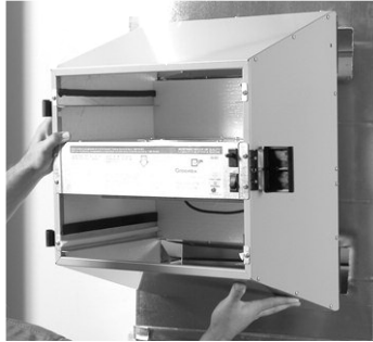
figure 2.3a - Align unit into place.
